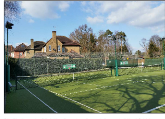
Site Photograph of Existing Boundary Fence Adjacent to 2 Northfield Avenue
